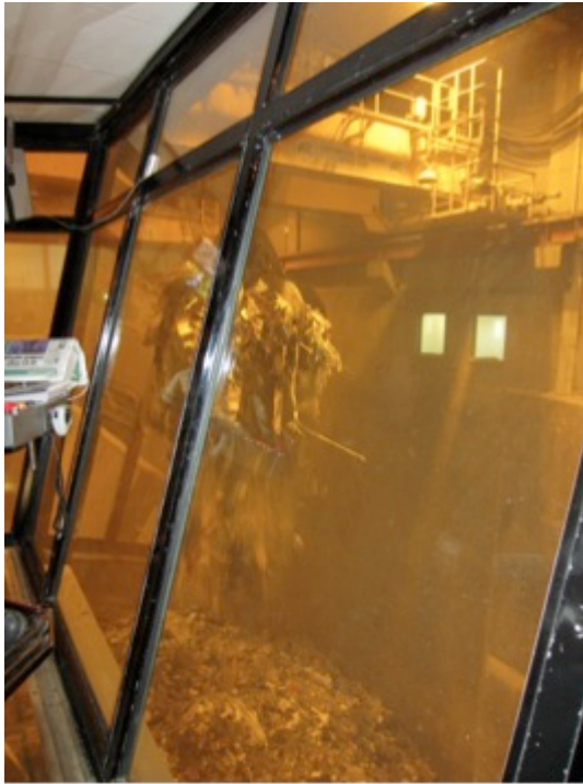
Figure 8. Crane operators and the crane at waste incinerator
