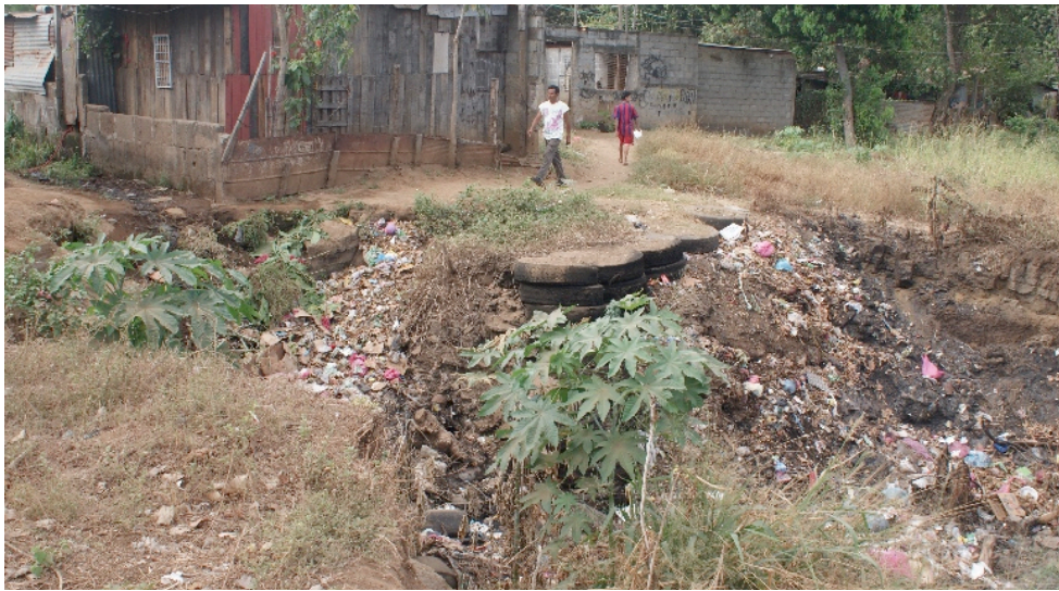
Figure 12. Riverbanks with waste.
