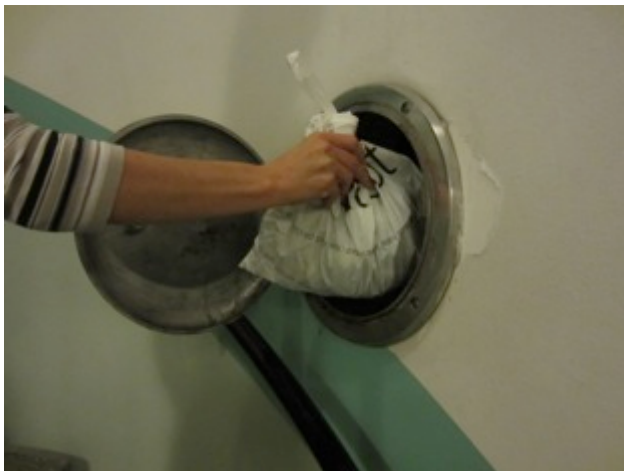
Figure 3. Waste vacuum system
